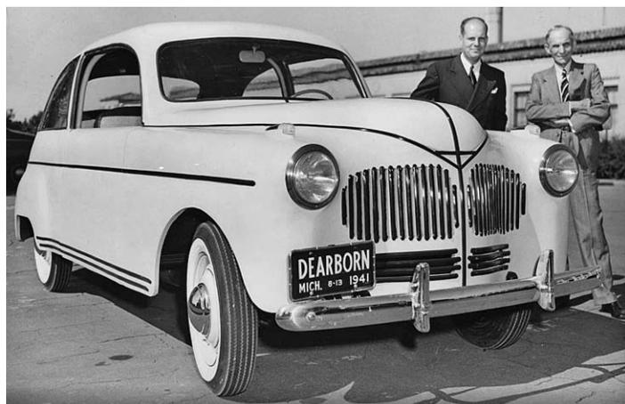
Robert Boyer, a chemist, oversaw a series of experiments at Greenfield Village’s Soybean Laboratory. The undertaking resulted in this plastic-bodied car. Henry Ford had a strong interest in plastic automobile parts. Always partial to projects combining industry with agriculture, Ford hoped plastic made from soybeans might be developed into a safe, strong substitute for traditional metals. “
